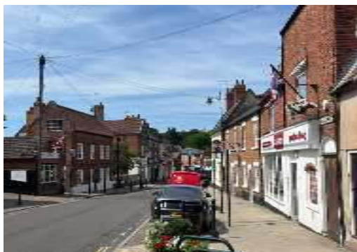
Figure 60: Varied rooflines example within Southwell
